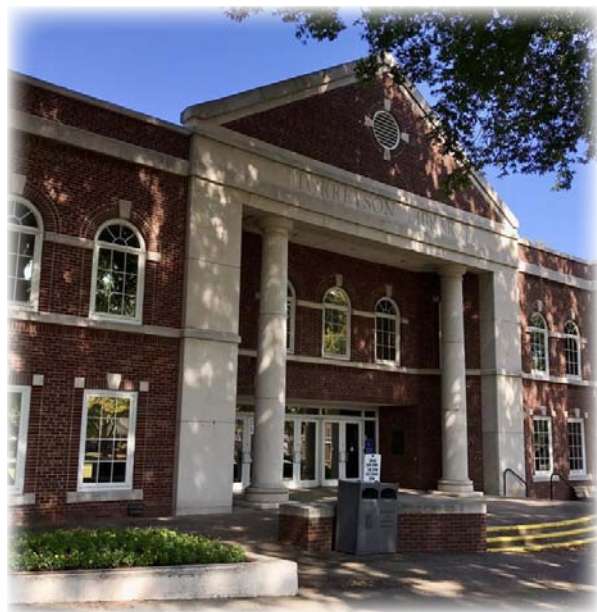
Torryson Library at University of Central Arkansas.
