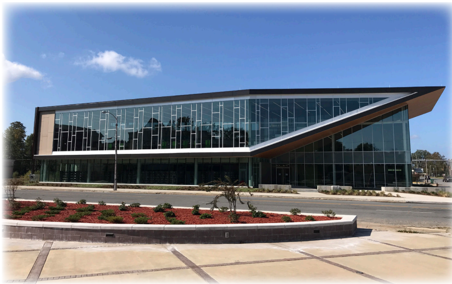
Pine Bluff/Jefferson County new Main Library. To read more, see pg. 8.
